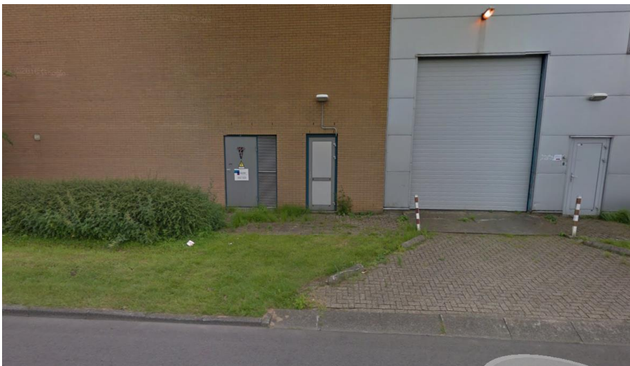
2: trafo Liander (in pandig)
